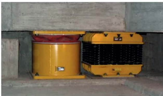
a) viscous damper and spring (BCS elements)
